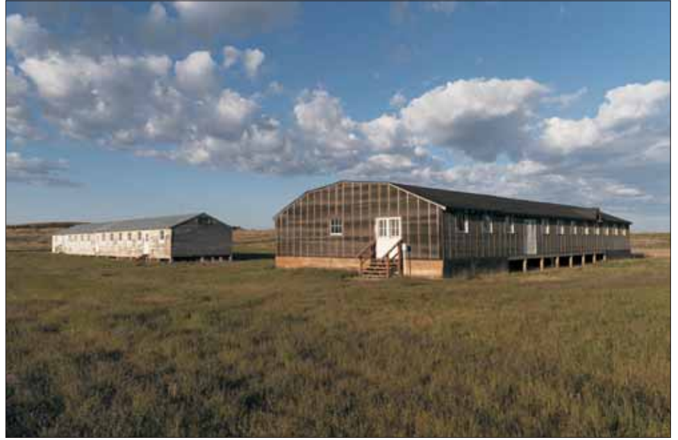
MINIDOKA ON OUR MINDS. The Block 22 barracks are seen at the Minidoka National Historic Site. “Minidoka on Our Minds,” an exhibit celebrating 25 years of preservation of the Minidoka National Historic Site, where many Nikkei from Oregon and Washington were forcibly incarcerated during World War II, is on view through June 14 at the Japanese American Museum of Oregon in northwest Portland. (Photo/Stan Honda, courtesy of the National Park Service)
